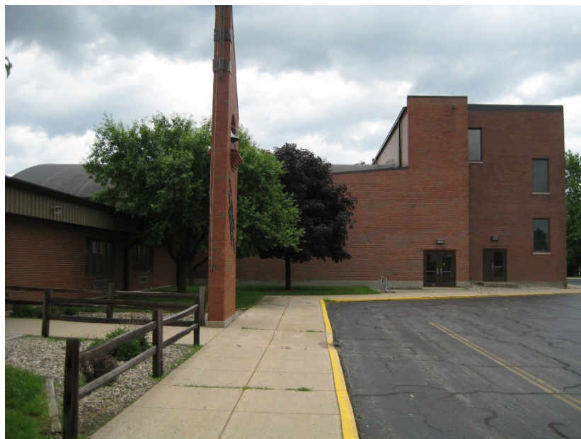
Former Reynolds Elementary School, proposed location of the White County Institute for Leadership in Alternative Energy.
